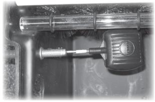
WFS37 — Install the autofill in the back wall of the skimmer by drilling a <sup>3</sup>/<sub>4</sub>" hole 3" down from the top of the skimmer. The auto fill is usually located in the back wall of the skimmer in the pump chamber (see photo).
